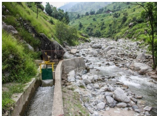
Figure 2. Intake of under construction MMHP
