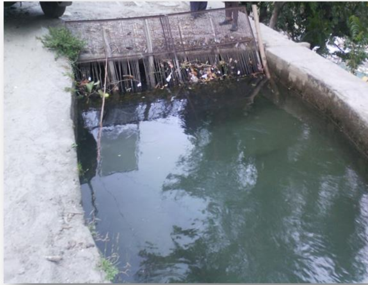
Figure 6. A Fore bay tank of an MMHP
