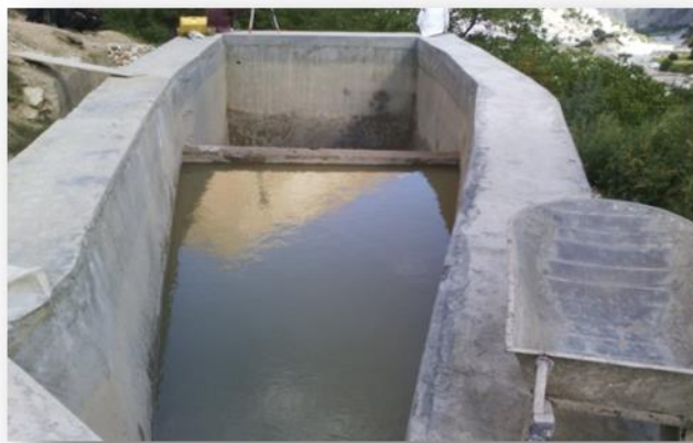
Figure 5. The setting basin of an MMHP
