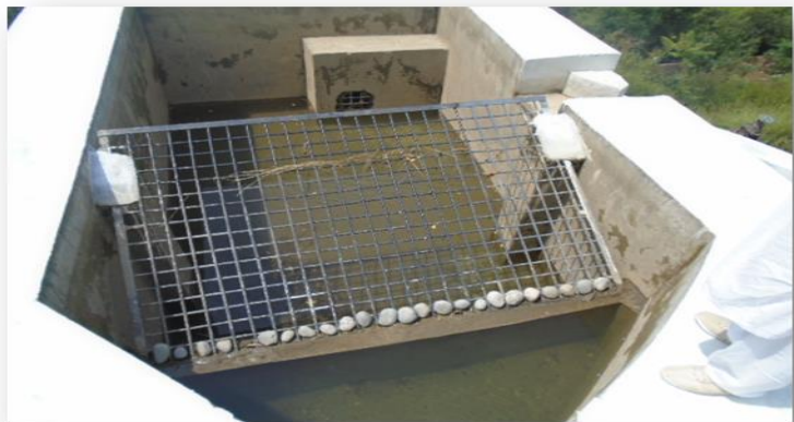
Figure 7. A Trash Rack aerial view of a functional MHP
