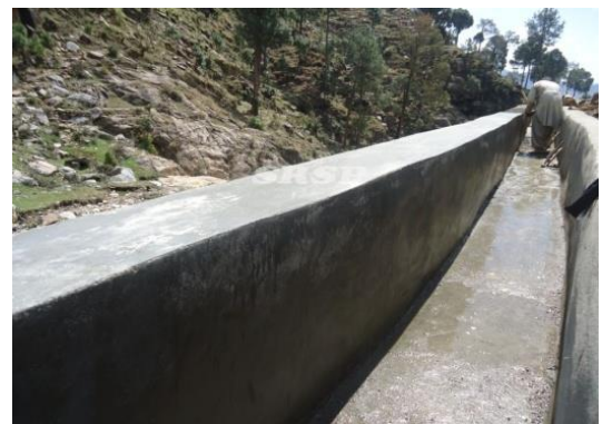
Figure 4. The channel of an under construction MHP
